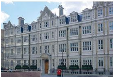
Central Court, 25 Southampton Bldgs - WC2A
